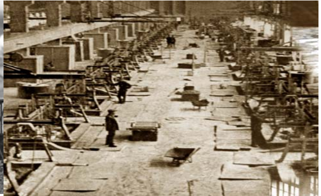
Figure 5. Volkhov Aluminium Smelter. Potroom №1
